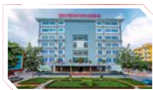
Hung Ha General Hospital Project
