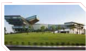
Marriott Hanoi Project
