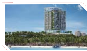
Movenpick Ha Long Project
