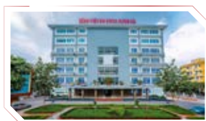
Hung Ha General Hospital Project
