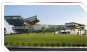
Marriott Hanoi Project
