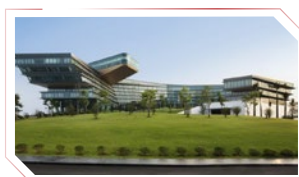
Marriott Hanoi Project
