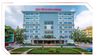
Hung Ha General Hospital Project
