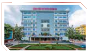
Hung Ha General Hospital Project
