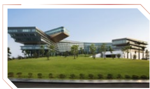
Marriott Hanoi Project
