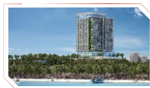
Movenpick Ha Long Project
