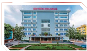
Hung Ha General Hospital Project
